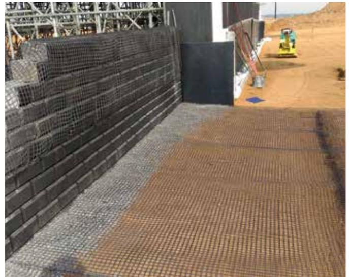
In the Active System the earth reinforced block and facing wall create an inseparable structure, i.e. reinforcements work in the earth reinforced block and in the modular block facing.
